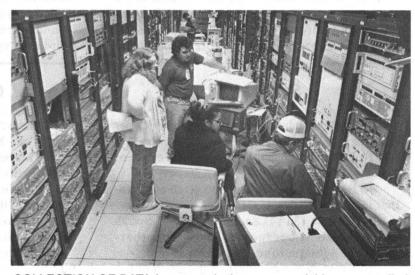
COLLECTION OF DATA from tests is the purpose of this room, staffed by employees of EG&G under technical supervision by Sandia. Most data is now carried out the entrance of the tunnel by fiber optic cables and transmitted several miles for central collection. Formerly, it went vertically through drill-holes to the mesa top for recording on equipment housed in trailers.
